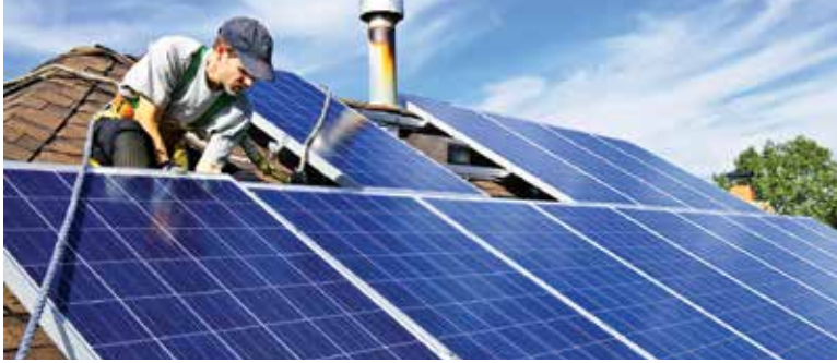
Solar panels on this roof collect the sun's rays to create electricity.
